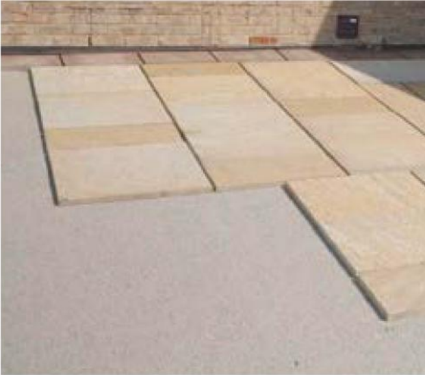
TYPICAL DRY-LAID NATURAL STONE PATIO/WALKWAY
